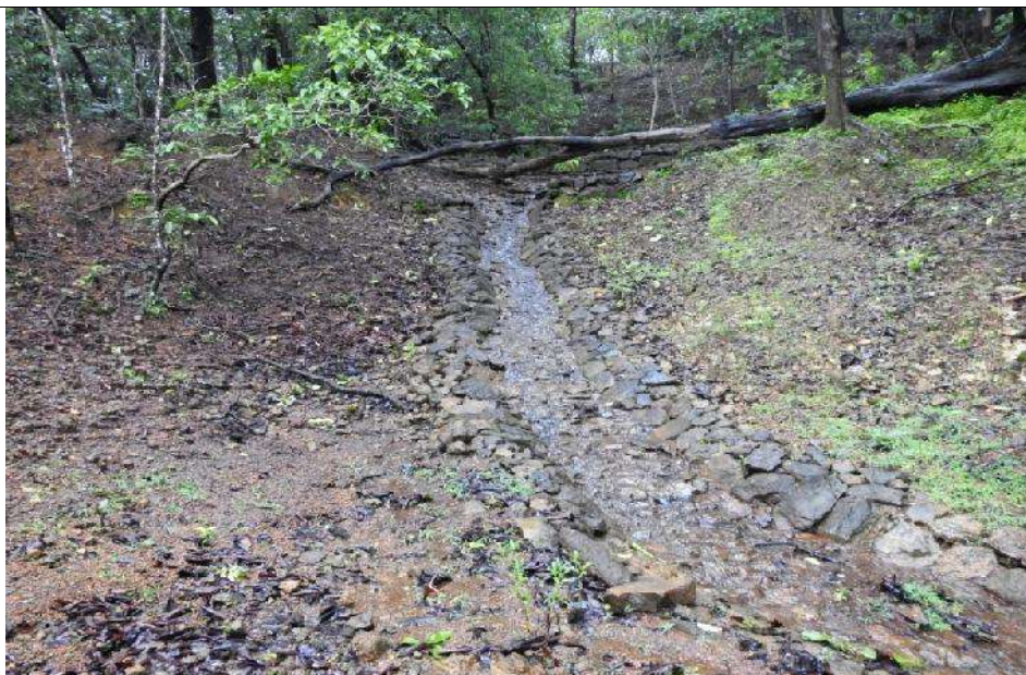
Fig. 3.8: Trenches made for water recharging
